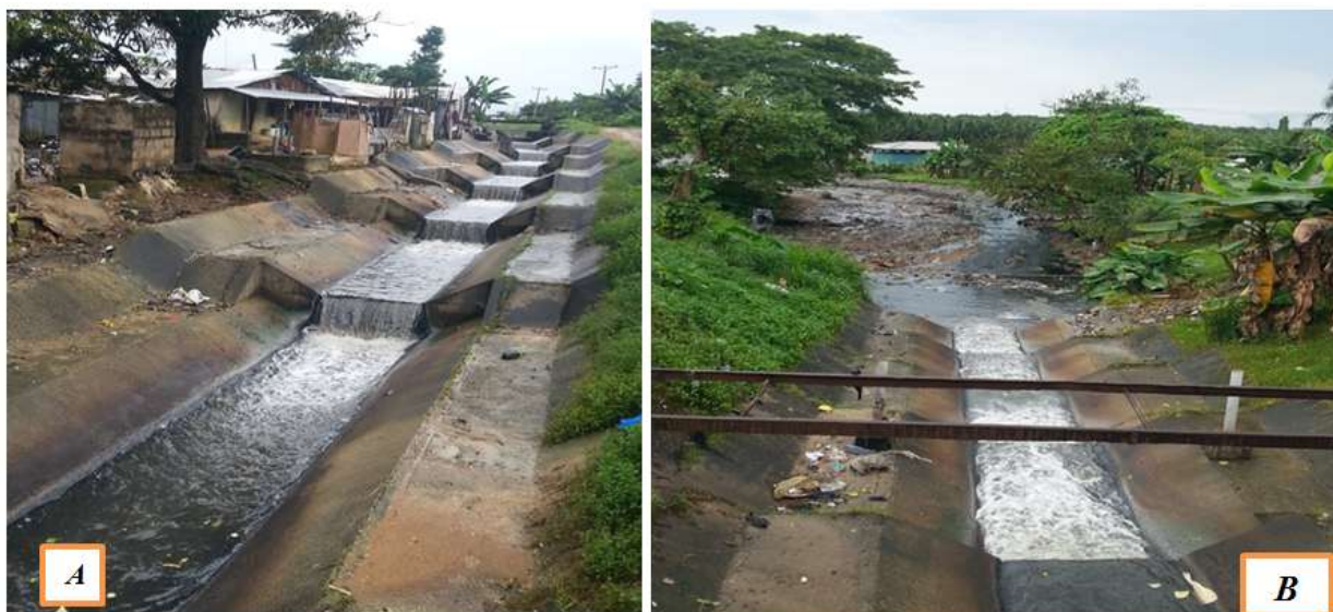
Fig-1: Picture of PHRC effluent paved drainage through Ekerekana community (A) discharging into a receptacle (B) – a creel in Ekerekana community, which directly flows into Okochiri River.
